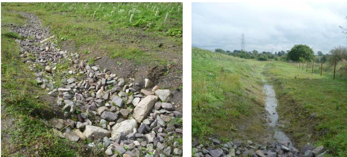
**Figure 11.** South-west tip, armoured drain with sill (left) and merging into swale on west boundary (right) on 9/9/11
