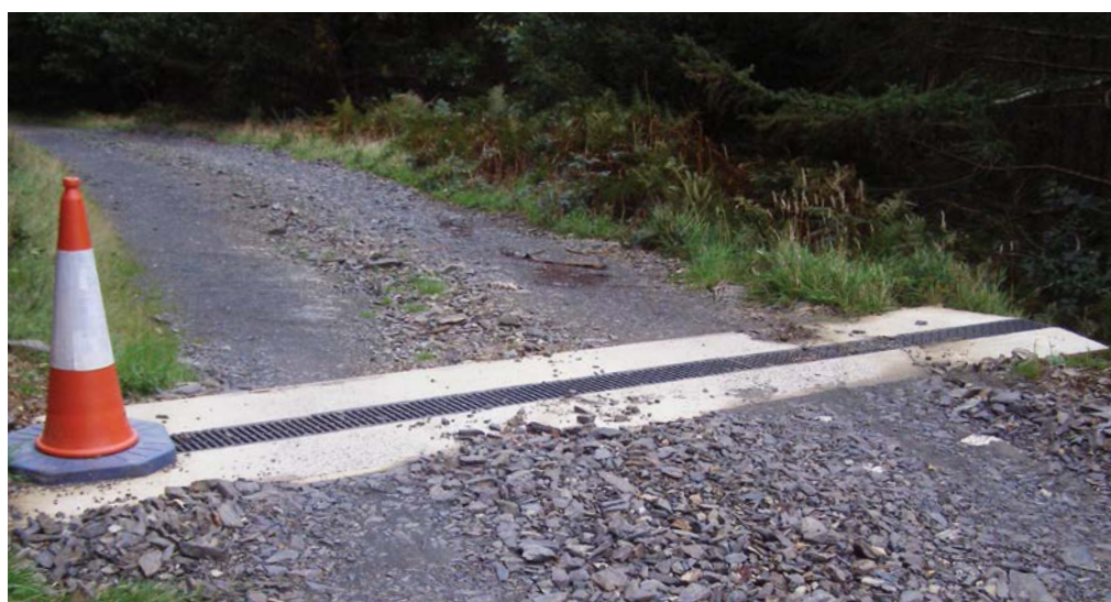
Figure 16 Install regularly spaced culverts or cross-gutters to split and reduce road run-off. These will need to be maintained to remain effective.
