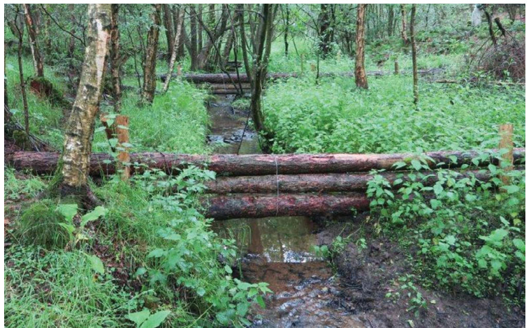
Figure 23 Closely spaced dams as shown here are likely to be drowned out by the backing-up of floodwaters, reducing their overall effectiveness.
