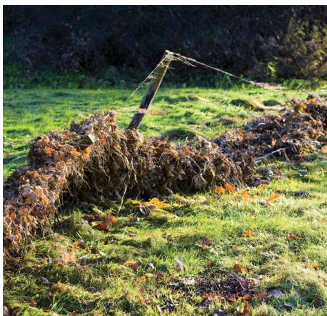
Figure 9 Mesh fencing can easily fail as a result of trapping leaf litter and woody material during flood events.
