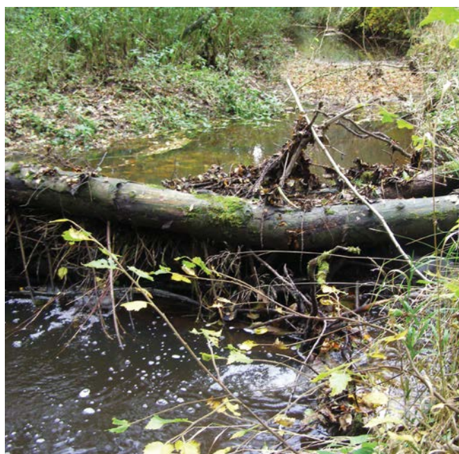
Figure 21 Leaky woody dams are most effective at high flow, when they hold back and push floodwaters onto the floodplain, increasing flood storage (left). However, 'weak' dams can be washed out at high flows (right), where the top log has broken and is likely to fail during the next flood event.
