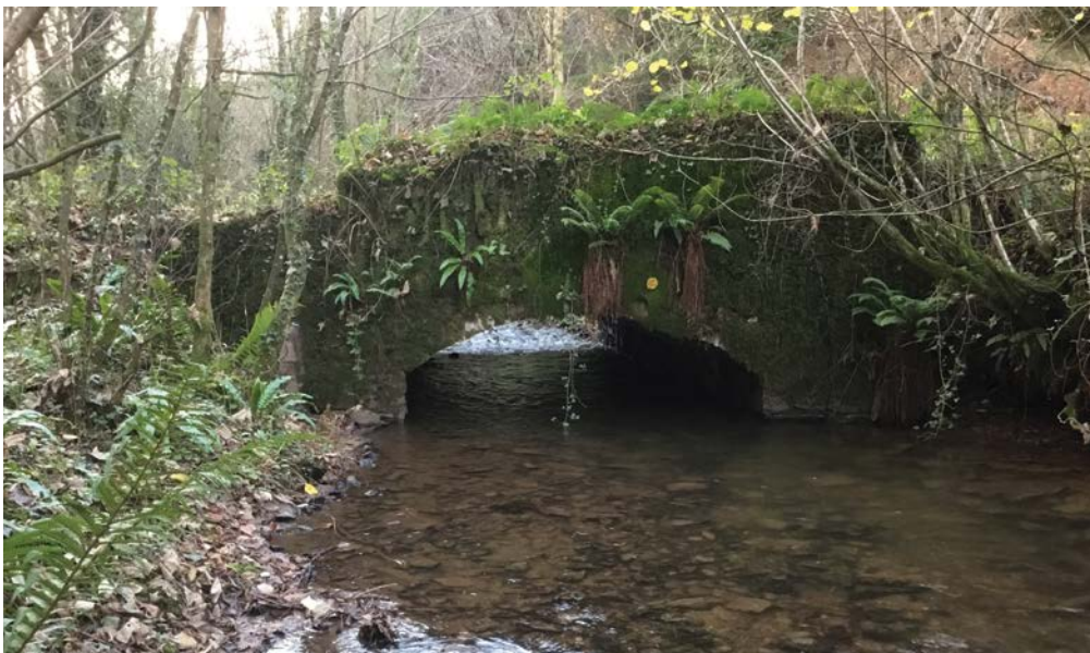
Figure 8 Low bridges constrain and back up flood flows, reducing the effectiveness of local upstream planting.
