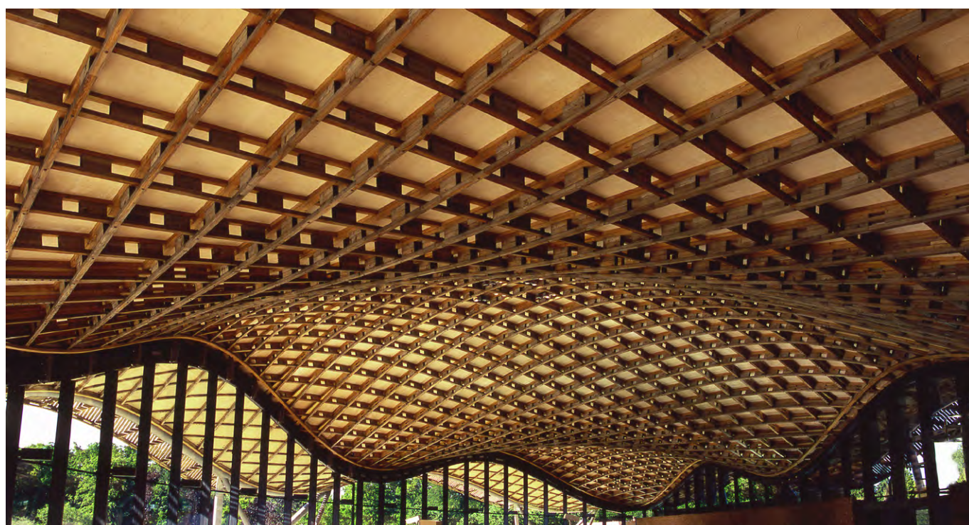
Figure 25 Interior photograph of the Savill Building Visitor Centre in Windsor Great Park (Crown Estates) featuring a timber shell roof. The building was designed by Glen Howells Architects.
