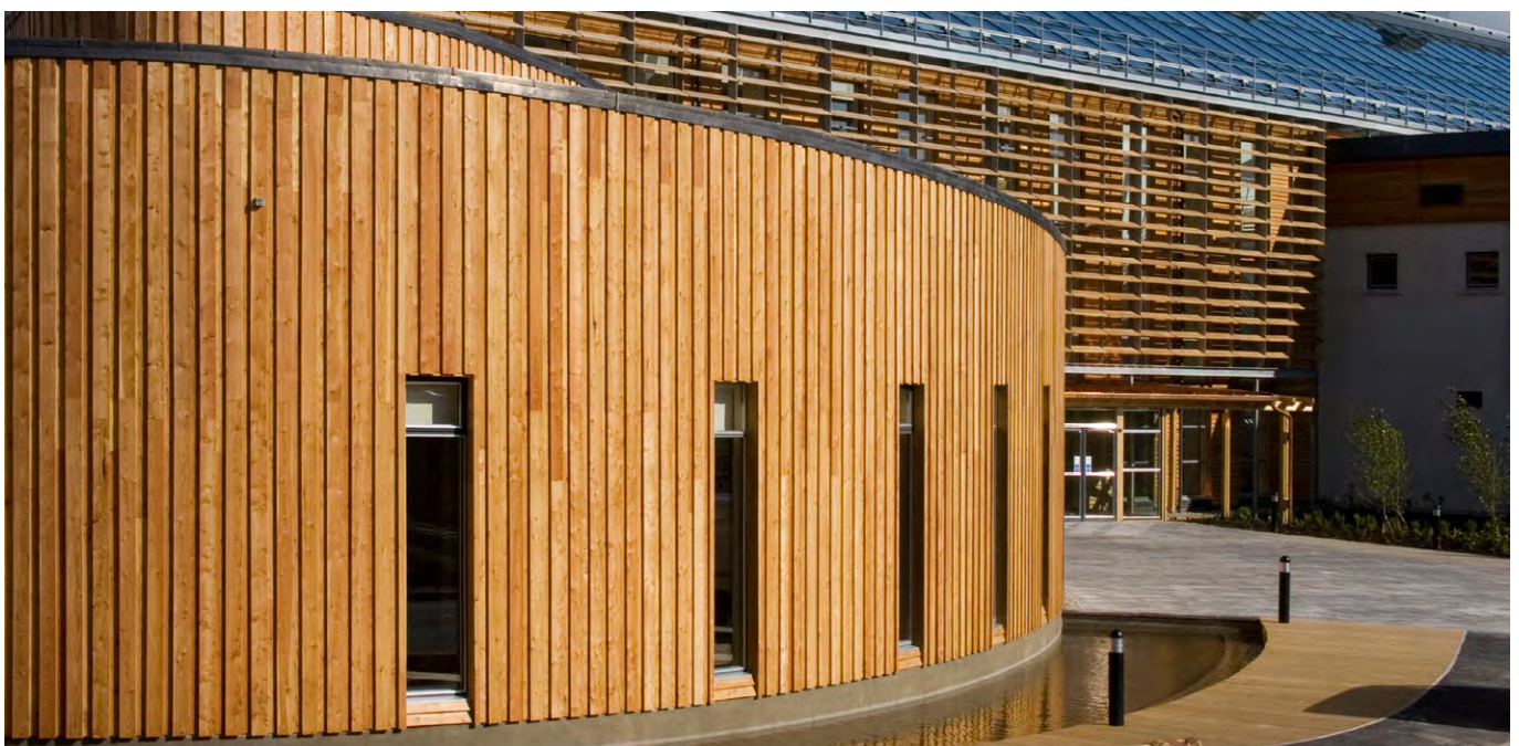
Figure 24 The headquarters for NatureScot in Inverness uses locally sourced larch for the external cladding and solar shading.
