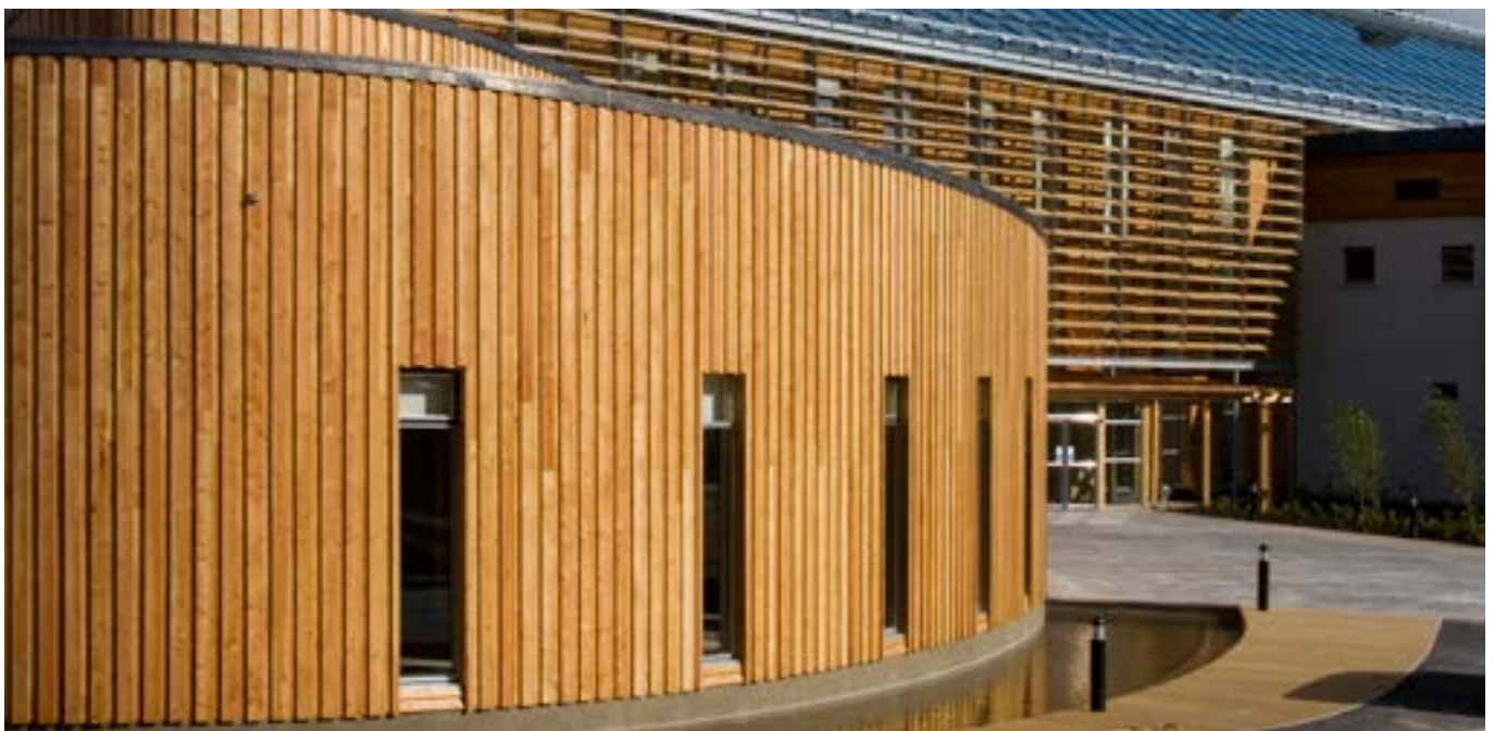
Figure 24 The headquarters for NatureScot in Inverness uses locally sourced larch for the external cladding and solar shading.
