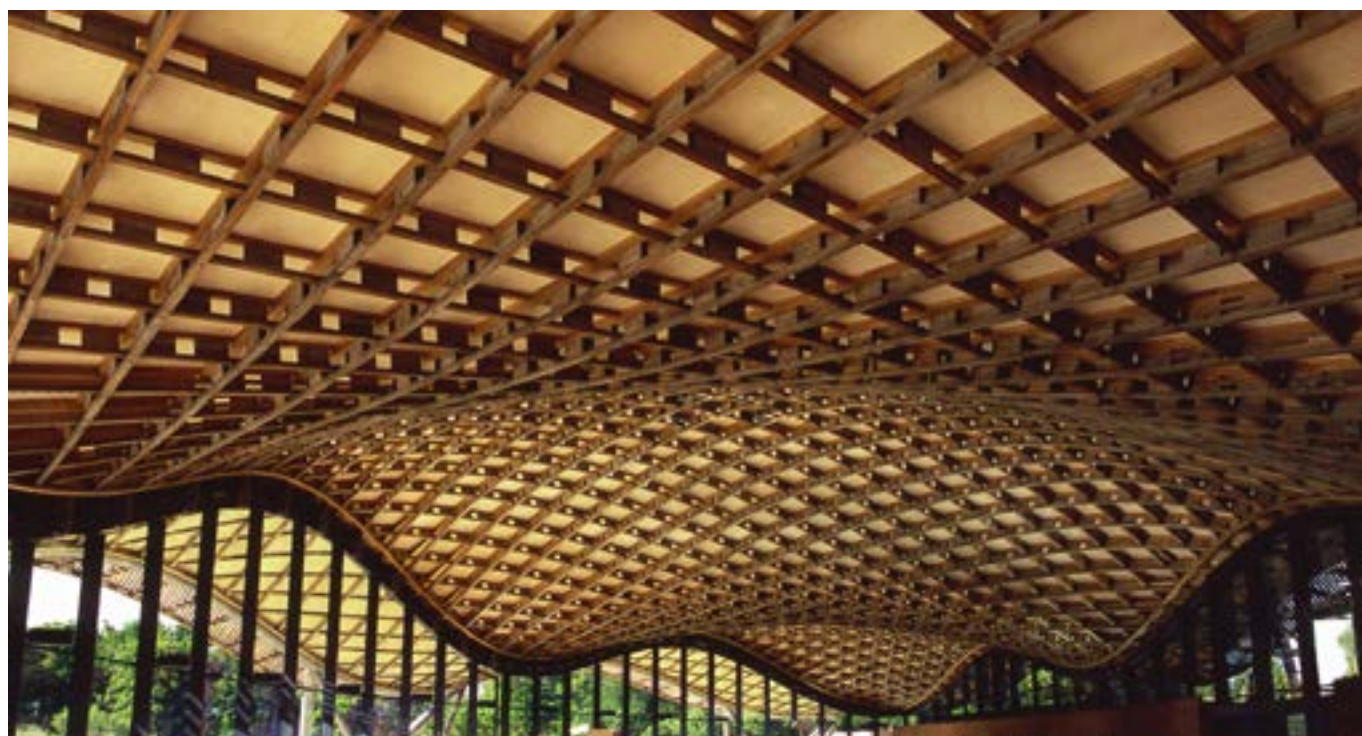
Figure 25 Interior photograph of the Savill Building Visitor Centre in Windsor Great Park (Crown Estates) featuring a timber shell roof. The building was designed by Glen Howells Architects.
