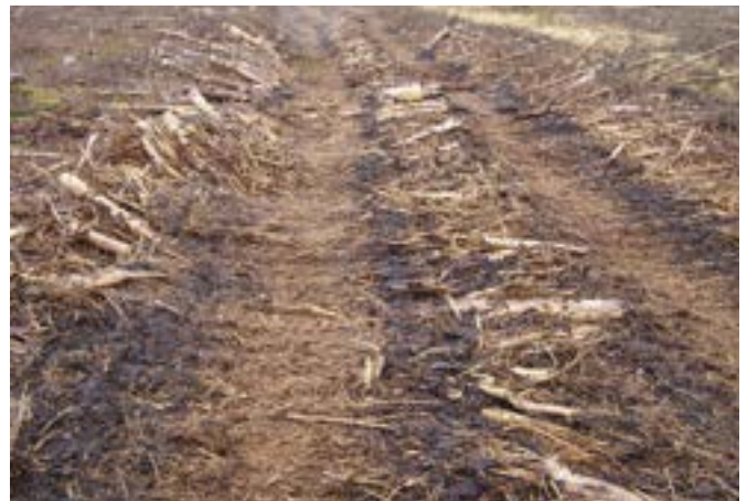
Figure 26 Logs plus brash may need to be used to protect very soft ground from harvesting damage.
