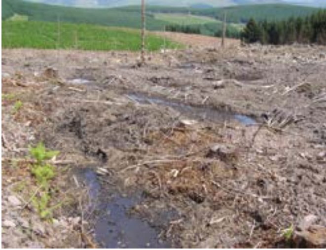
Figure 27 At this site, failure to respect watercourses has resulted in significant soil disturbance and siltation.
