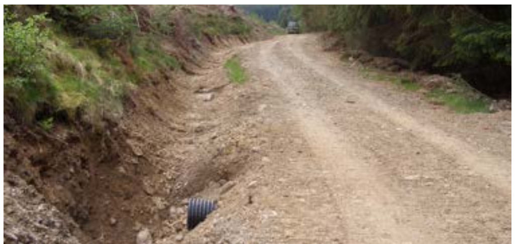
Figure 15 Install regular culverts to manage road drainage.
