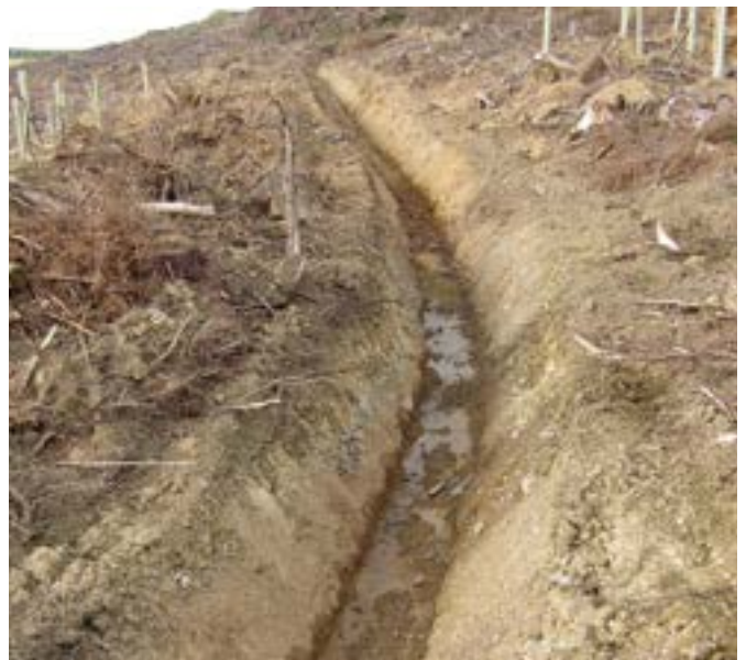
Figure 8 An example of a well-designed cut-off drain controlling restock site run-off.
