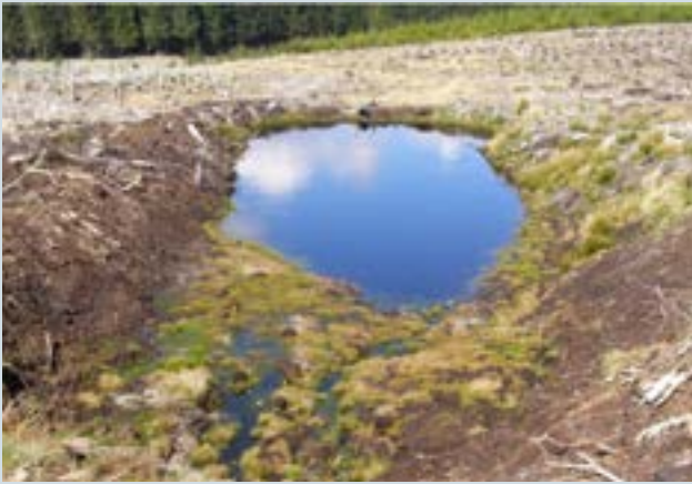
Figure 33a Large silt traps can hold more water and help to settle finer sediment but need care to avoid washout of bund, especially at outlet at high flow.
