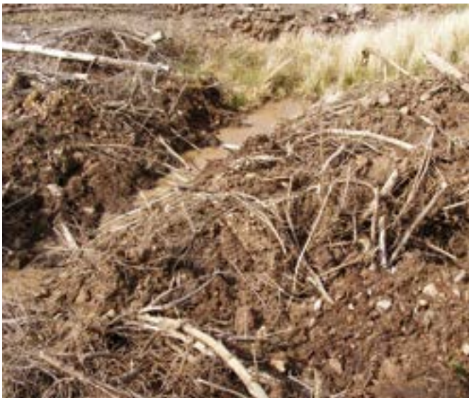
Figure 4 Excessive soil disturbance can lead to sediment-laden run-off and should be avoided. It isn't enough to rely on buffer areas to protect watercourses.
