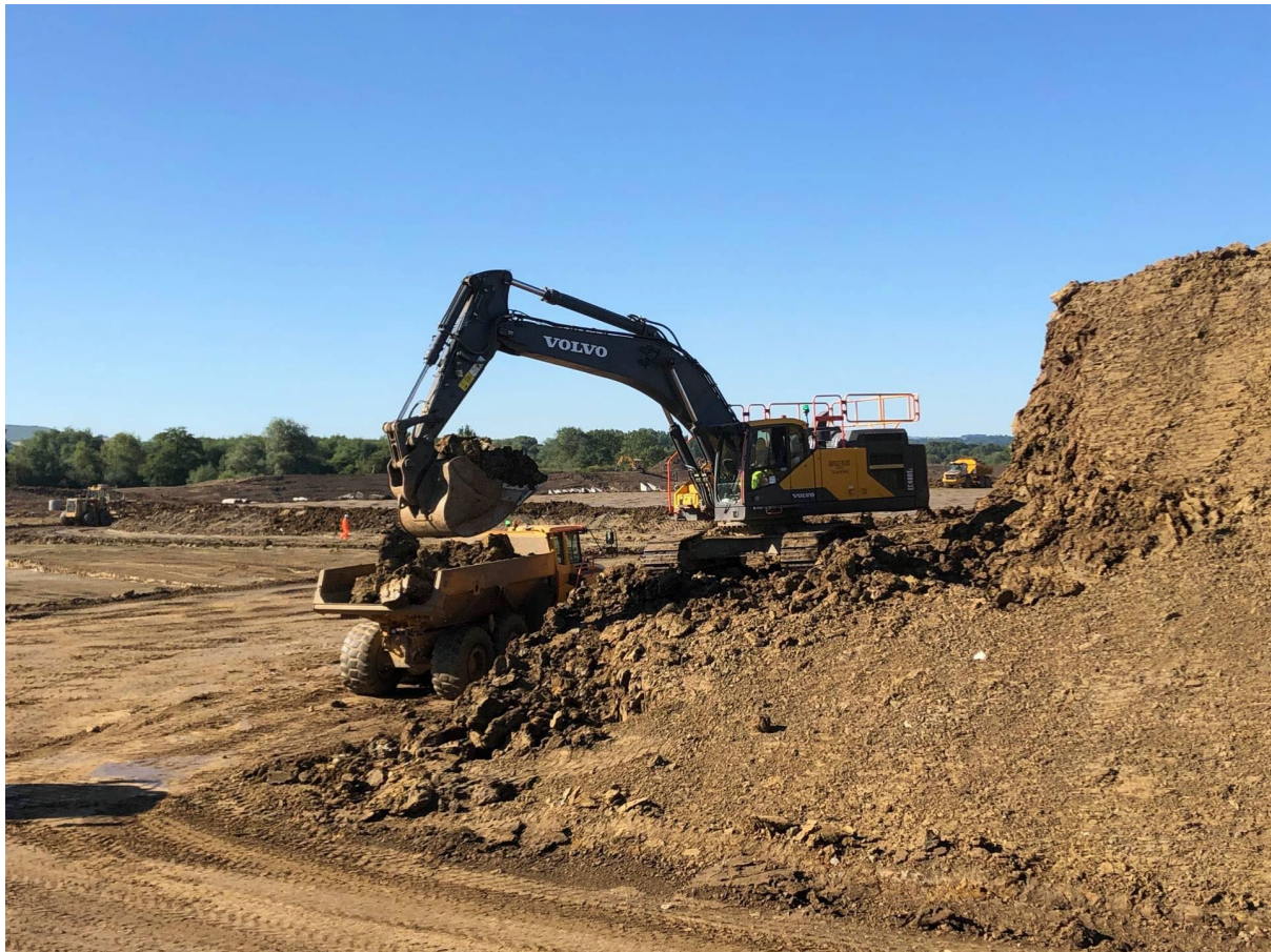
(photo: Tim O'Hare Associates)
